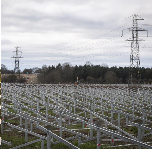
Construction ongoing at Tiln, Nottinghamshire
