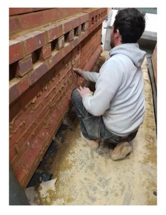
Plate 13 – Finishing of Mortar Joint
