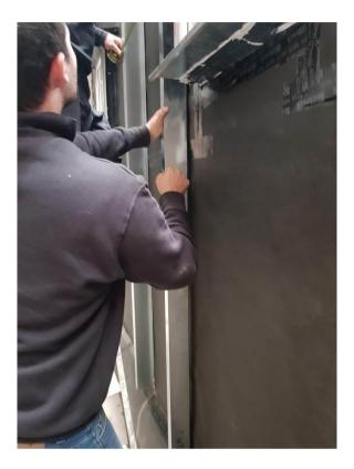
Plate 8 – Installation of Zed Rails
