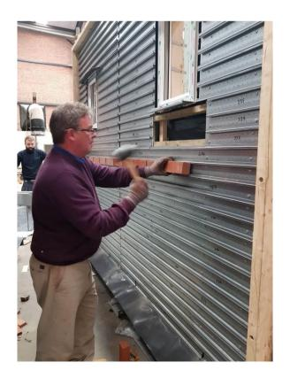
Plate 11 – Installation of Brick Slips
