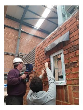
Plate 12 – Application of Pointing Mortar
