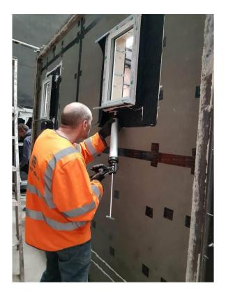
Plate 4 – View of the 'DPC Installed to Window Perimeter and Cement Particle Board
