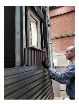
Plate 10 – Installation of Brick Rail
