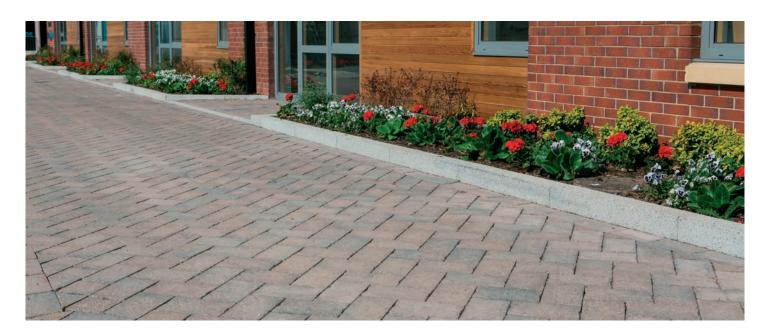
Installing a permeable paving sustainable urban drainage system (SUDS) eradicates surface pooling and puddles while allowing rainwater to be harvested and reused. Its use can reduce the risk of flooding and help control the amount of water that enters the drainage infrastructure.
