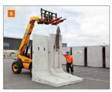
This is a lifting operation and is covered by LOLER, as such a competent slinger / AP is required to manage the lift. All non-essential operatives are to be excluded from the vicinity of the lift.
