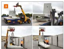
The QuickLift system has been developed to ensure that no additional lifting equippeded other than convention I chains and hooks for the three lifting points. Unlike many other systems we have no hidden costs for expensive lifting gear.
