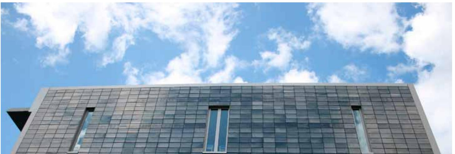
Forterra's Red Bank Lockclad terracotta tiles provide a ventilated rain screen that offers architects a durable and low maintenance finish.
