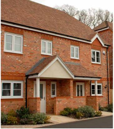
The South Down Multi is a 'true' tumbled product as it is tumbled in the green state so as to give 'soft' tumbled edges. The contrasting brick on this particular development is the Atherstone Red, a plain red stock brick, which has been used for detailing on the dwarf walls, above the windows and below the roofline.
